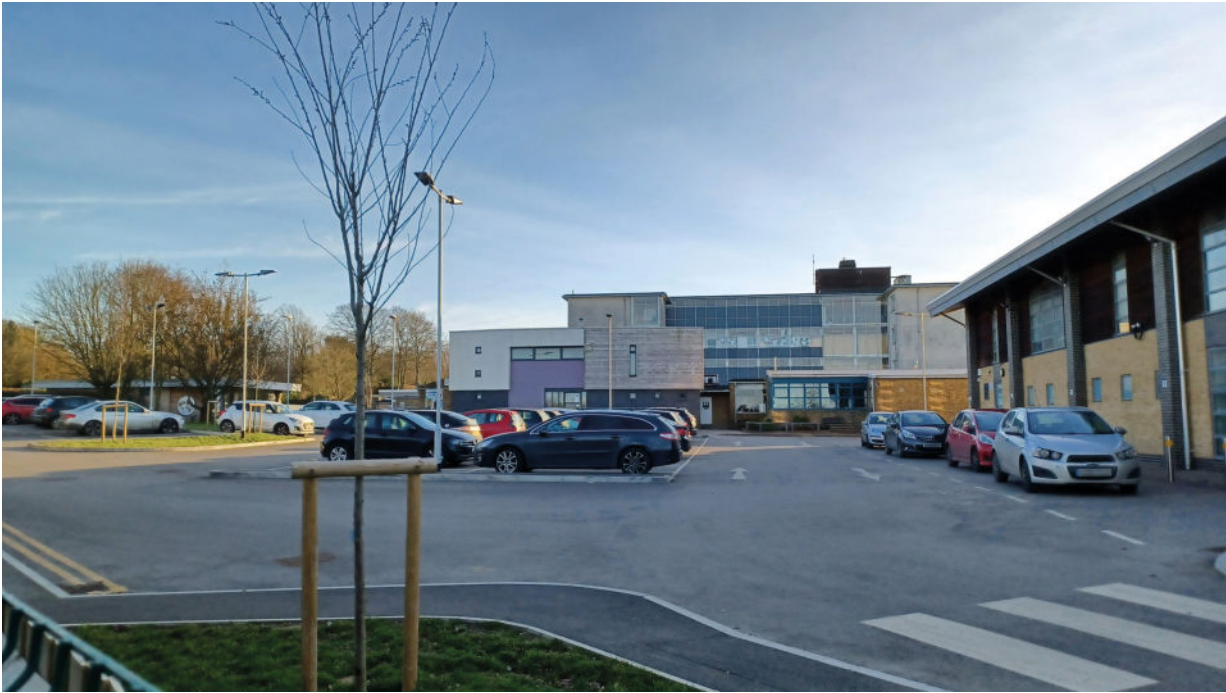
Photograph 3 – View showing existing school buildings
