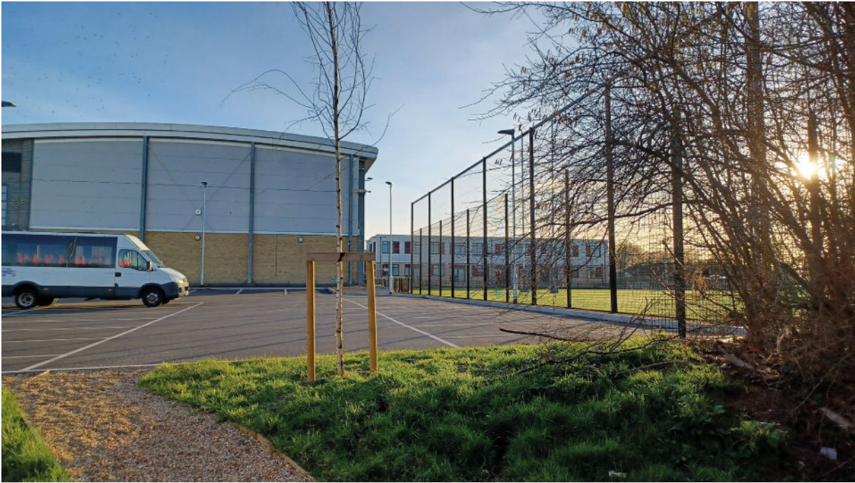
Photograph 1 – View across the site from the footpath looking towards the sports hall
